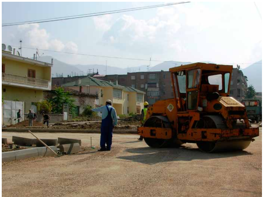
Photo: Road construction began in Korça's Neighborhood 15. Credit: USAID/LGPA.
